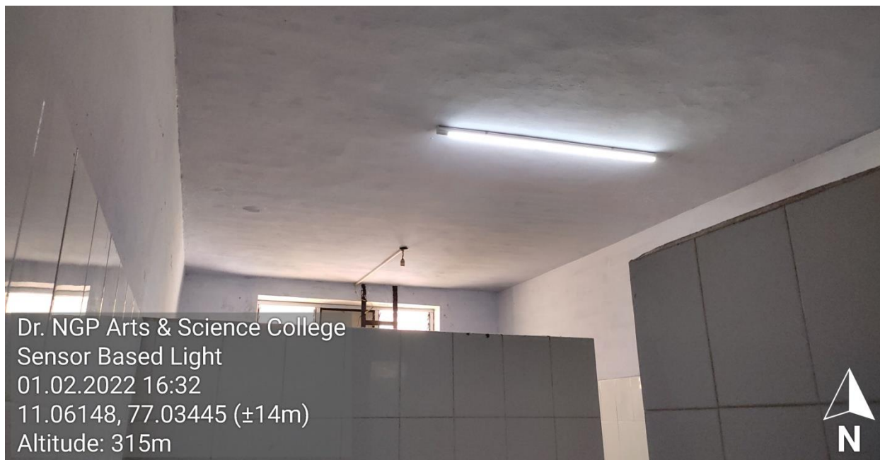
Sensor based light (Dim mode) fitted in staff rest room at A1 Block
